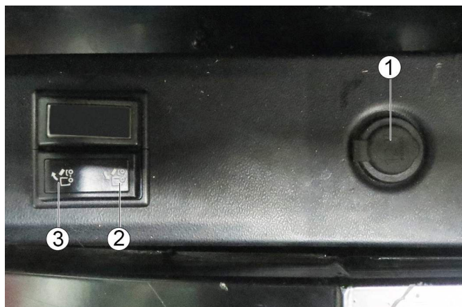
Waste container controls
